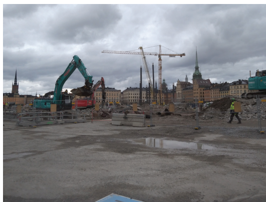
Figure 4. Slussen area under reconstruction in spring 2021
