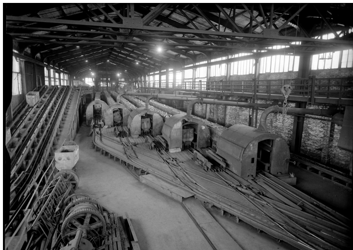
Figure 2. View into a shaft hall with wagon circulation, Kaiserstuhl 2 colliery, Dortmund, 1950s
